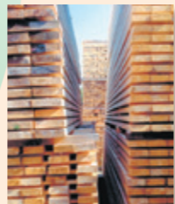
Construction materials storage site
